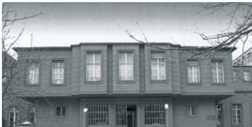
The former building of the Ministry of Commercial Affairs in Ankara
