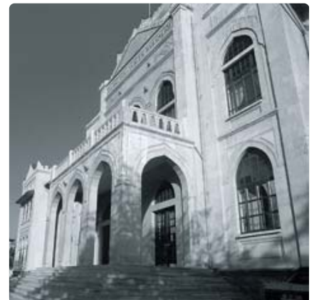
The former building of the Ministry of Customs and Monopoly
